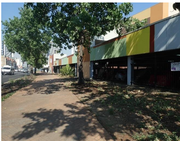
Figure 25 Western view along Terminus Street of the two-storey car park at the rear of 48-52 Scott Street.
