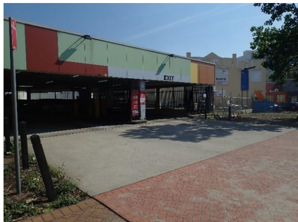
Figure 24 North-eastern view of Terminus Street entrance to the car park at rear of 48-52 Scott Street.
