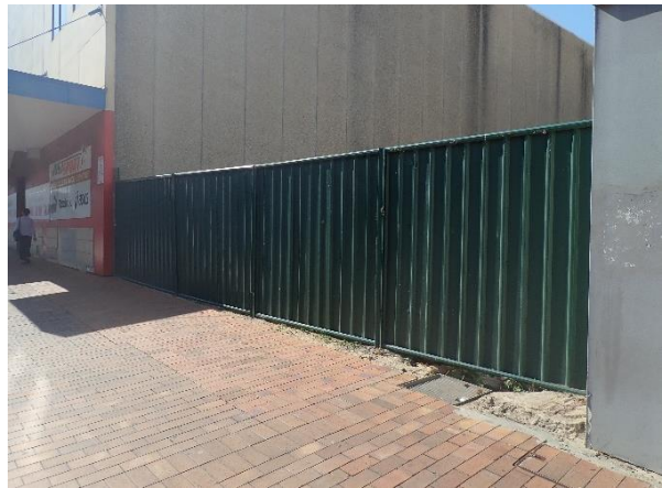
Figure 30 South-eastern view of Scott Street frontage of the vacant lot. A small portion of surviving footing was observed on the right-hand side. Refer next figure.
