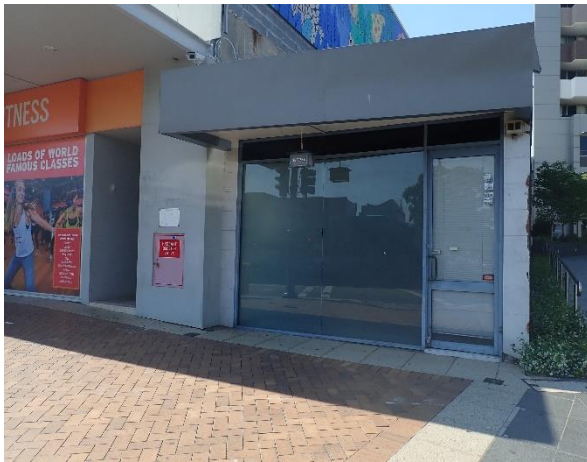
Figure 21 View to the south of 64 Scott Street.
