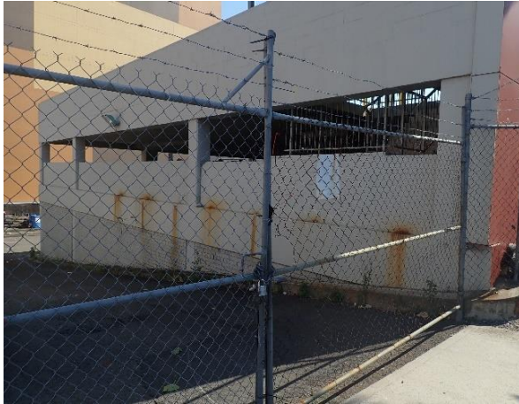
Figure 27 View to the north-east of western side of 48-52 Scott Street car park showing the change in level to the north.
