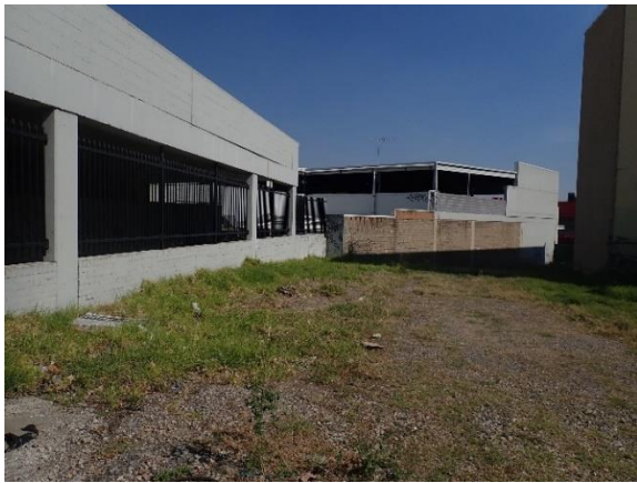
Figure 29 North-western view from Terminus Street down the vacant lot showing the change in level between Terminus Street and Scott Street as visible in the eastern face of the 48-52 Scott Street building and car park.
