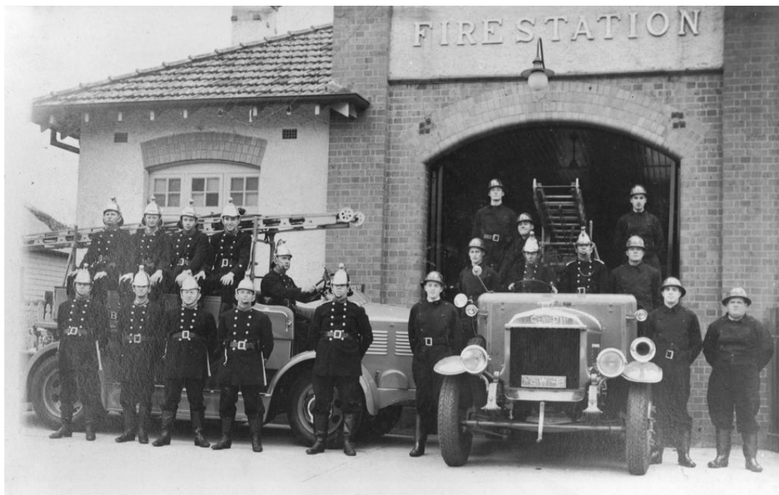
Figure 11 Liverpool Fire Brigade outside the Scott Street station in 1936. (Source: Liverpool City Council Library)
