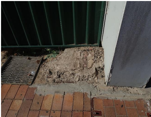
Figure 31 South facing image of surviving concrete and brick footing in the vacant lot.
