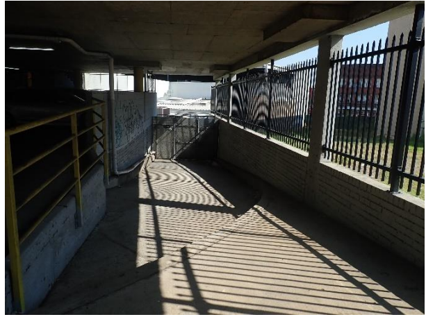
Figure 28 View to the north of eastern side of car park structure where a down ramp matches the slope observed on the western side (previous figure).
